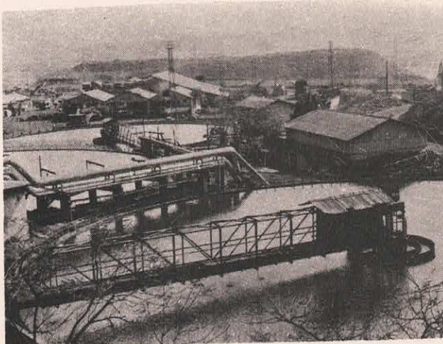
Effluents of Coal Washeries (SE/3)
