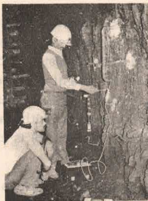
Measurement of pillar stress, strain and deformation deep depillaring (MT/9.3)
