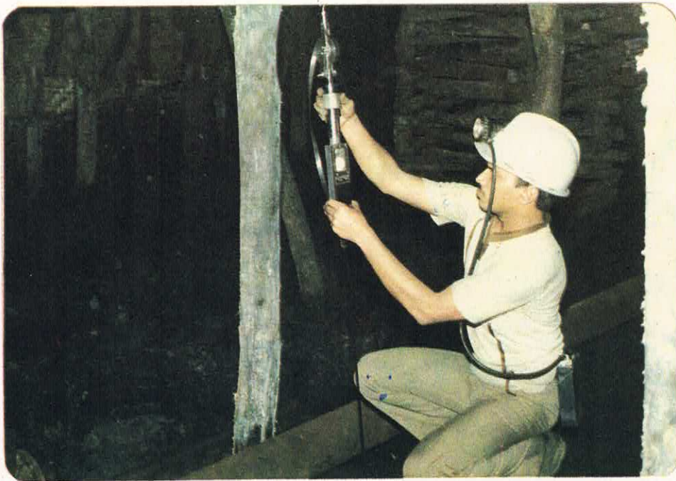
Roof convergence study along the goaf edge of conventional depillaring face. (MT/9.3)
